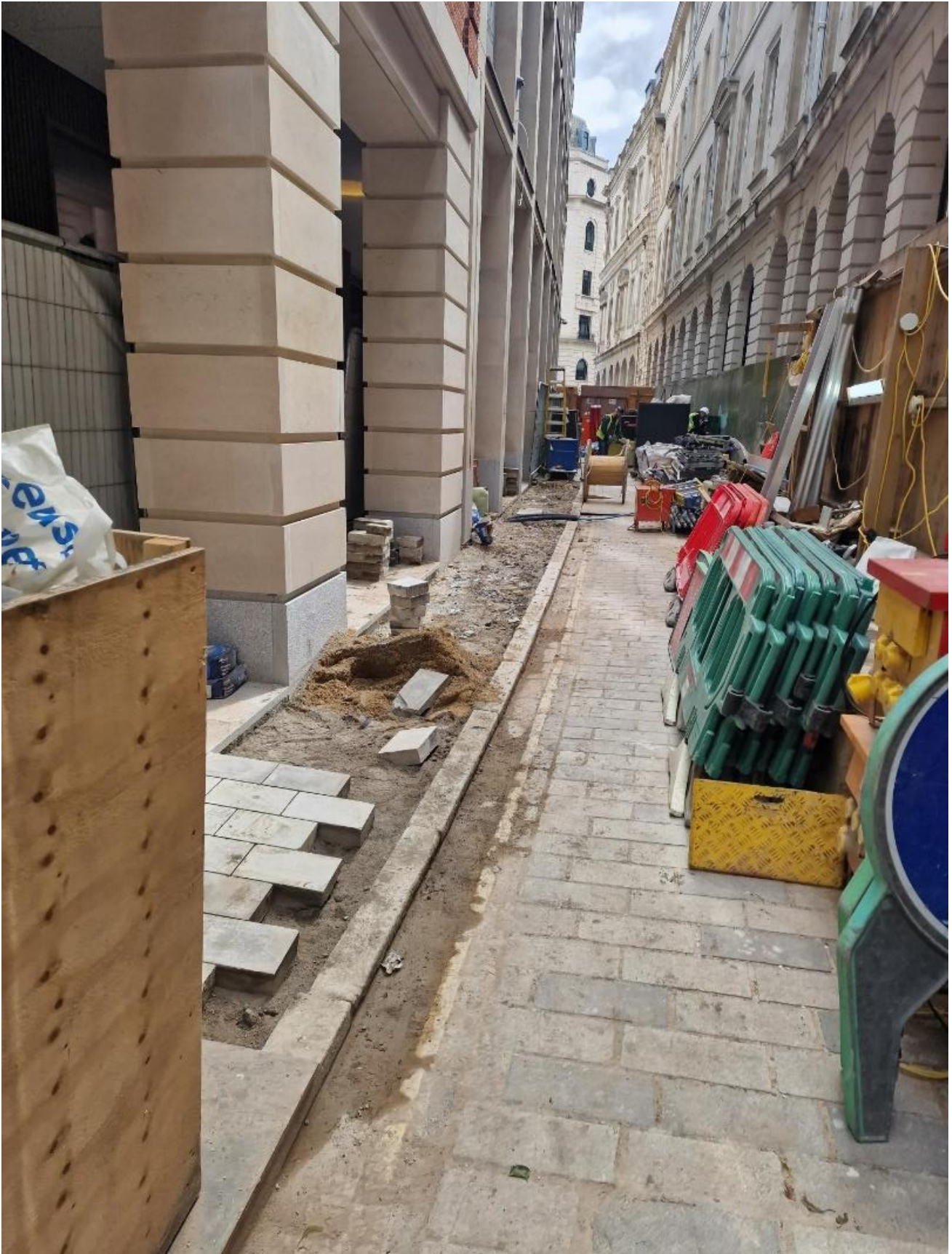
Ironmonger Lane | Hoarding to be removed to initiate improvements
